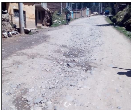
Figura 1. Carretera Huaraz–Paria–Willcahuain (zona Acovihay).
